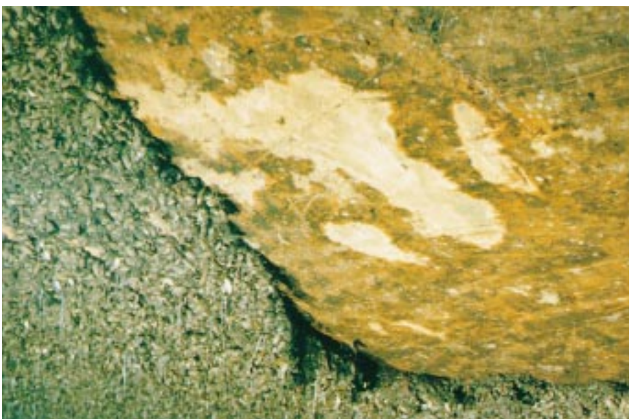
Thick fouling of barnacles, mussels and other shells on a ship's hull. The fouling must be removed by handscraping, followed by sweeping or blast cleaning where necessary. (Photograph courtesy Jotun Paints)
